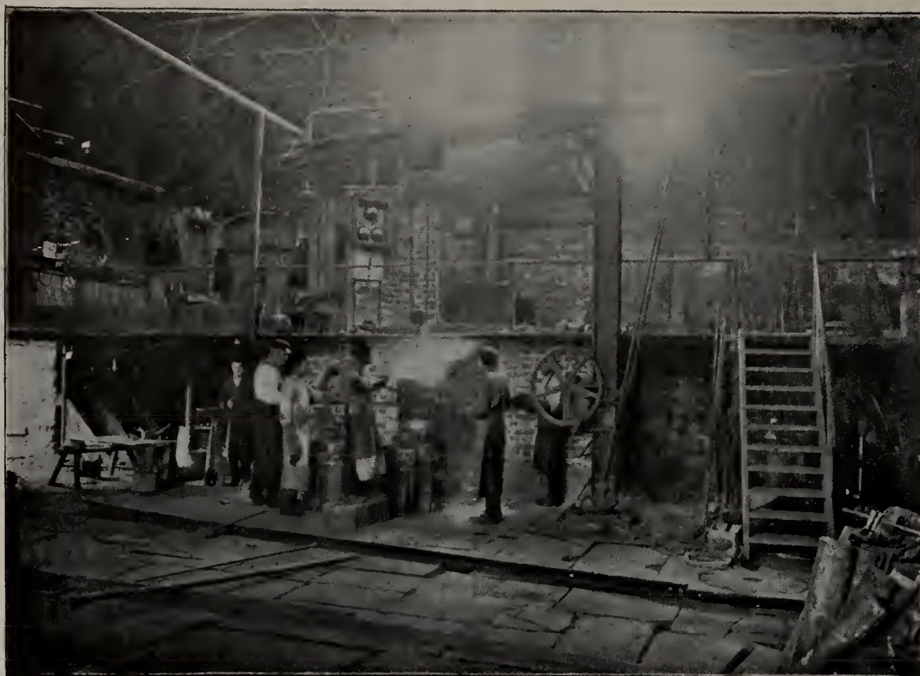
GENERAL VIEW OF KJELLIN ELECTRIC FURNACE AT GYSINGE, SWEDEN.
